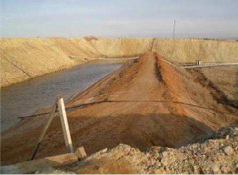
The solution percolates through the ore heap and is collected in the pregnant liquor ponds from where it is pumped to the sorption plant. The volume of an operating heap can vary from several hundred thousand to 1.5 million tons of ore. Typically, a heap is leached for one year while a new one is prepared to replace it.
