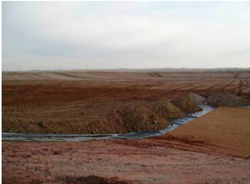
For heap leaching, the milled and classified ore is stockpiled in heaps on specially lined pads.
