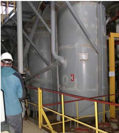
Photo 5 – Fluidized bed ion exchange columns
