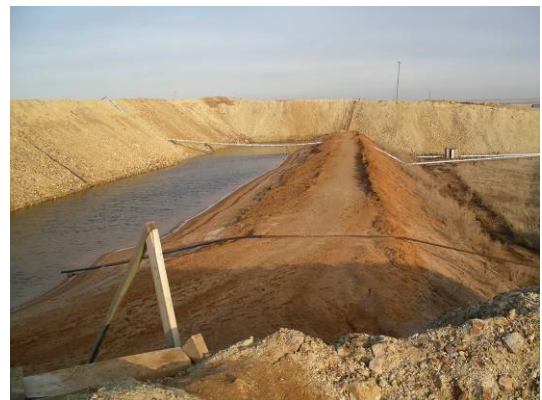
Photo 3 (right). Collector pond for the pregnant gold solution between the operating heap and dam
